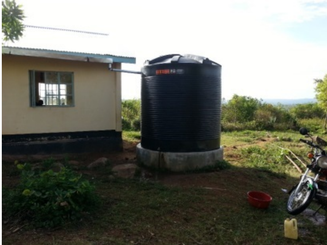
The recently installed rainwater tank at Nyabukemo Primary School (above) collected enough water to keep the school supplied throughout the extended dry season.
